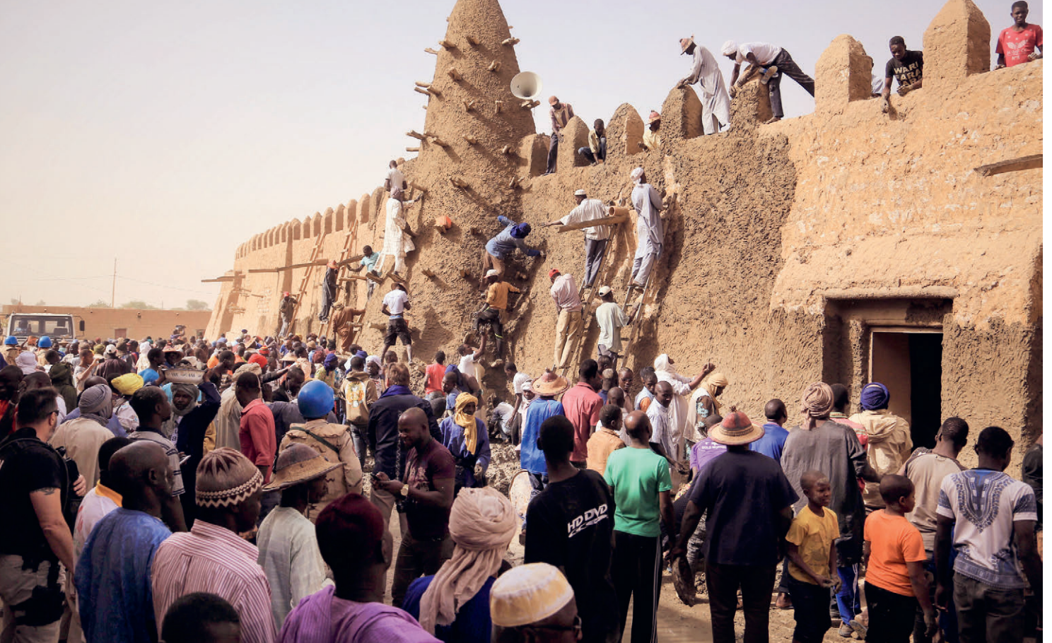
2 Reconstruction of the destroyed mausoleums of Timbuktu (Mali). © UNESCO (Photo: Bagayoko Modibo)
